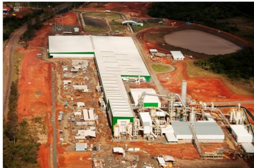
New MDP mill in Montenegro, Brazil
